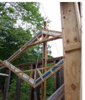
the trusses into the building, suspending them upside-down on the roof plate and pulling them upright using a rope run through the pulley. The trussed were big, heavy, and awkward and I was thrilled when David showed up and I was demoted to truss tie-er. I stood on the roof plate and when a truss was pulled upright I tied it to the support beam.
